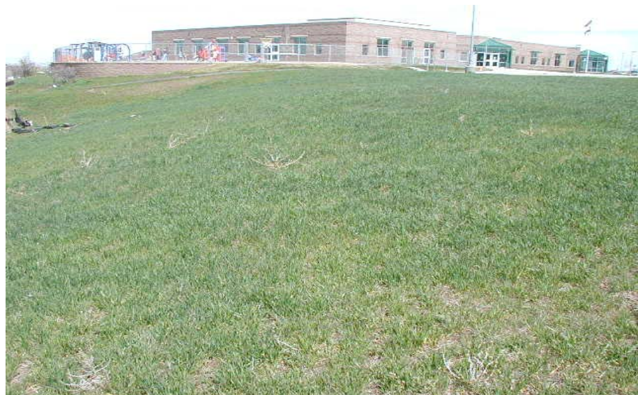
Full vegetation coverage is required prior to release of collateral.
