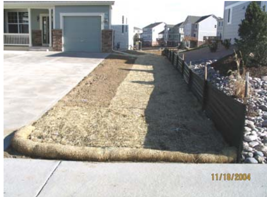
Homeowners are responsible for maintaining temporary erosion control measures on their property until permanent measures are implemented.
